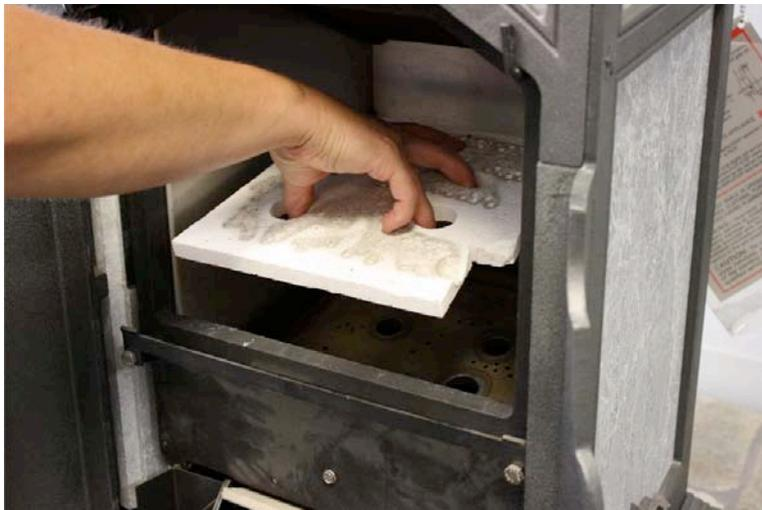
8. Clean any debris from the surface of the burner pan with a vacuum.
