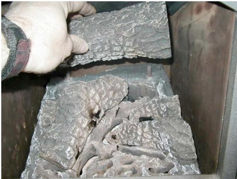
6. Carefully lift the log set out of the stove by the base of the log set. Do not pull up on any of the smaller logs as they will separate from the base.
